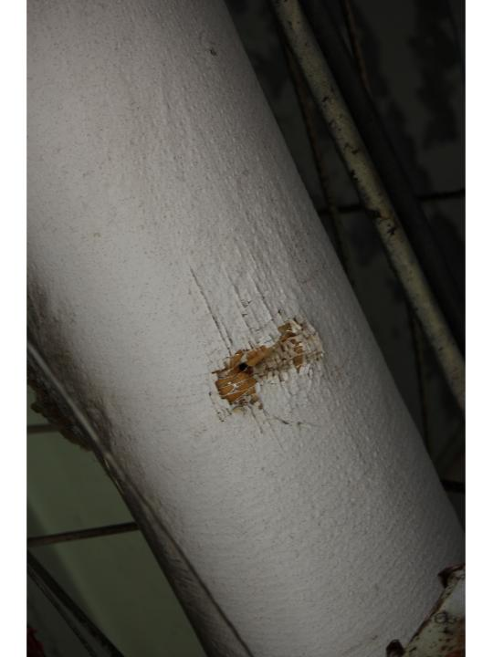
Asbestos abatement has not been completed. Degraded asbestos wrapped pipes are still in place.
