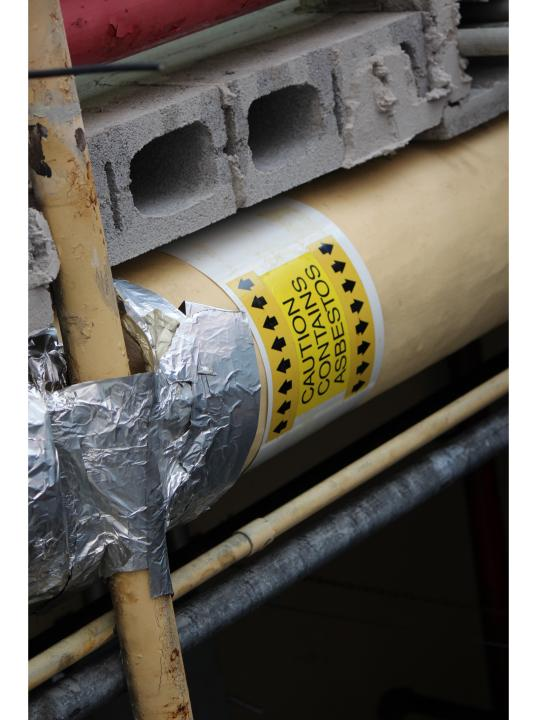
Asbestos wrapped pipes are damaged in many places.
