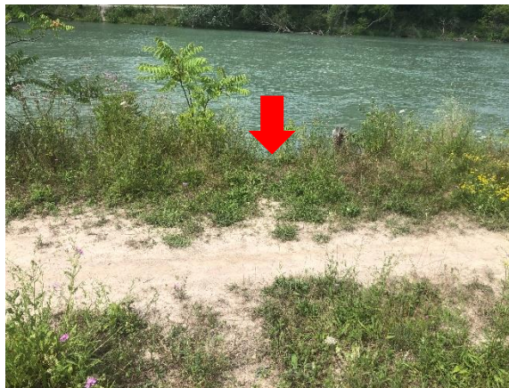
Plate 2: View of drainage channel in Plate 1 looking downslope to public bike path and drainage to TMC (red arrow). This channel shows bare soil with sparse plants in the general area, marked by blue arrow 1 on Figure 2.
