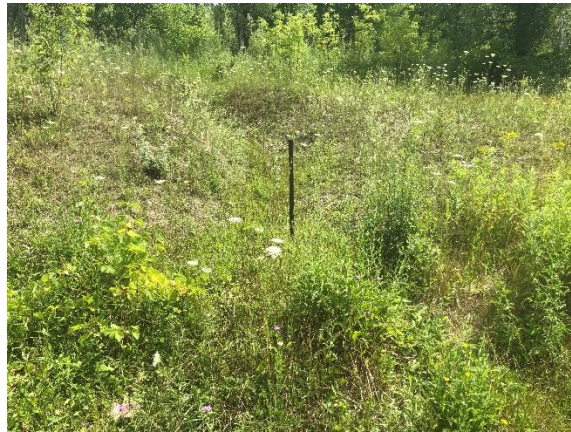
Plate 1: View of drainage channel looking upslope, marked with metal stake, that is about 1 m wide and about 0.5 m deep. Plants are sparse in the channel but grow along the edge, and thereby obscure the presence of bare soil in the channel. This channel corresponds to the location marked by blue arrow 1 in Figure 2.
